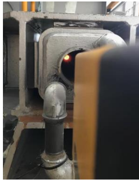
↳ Length & position measurement at furnace entry
